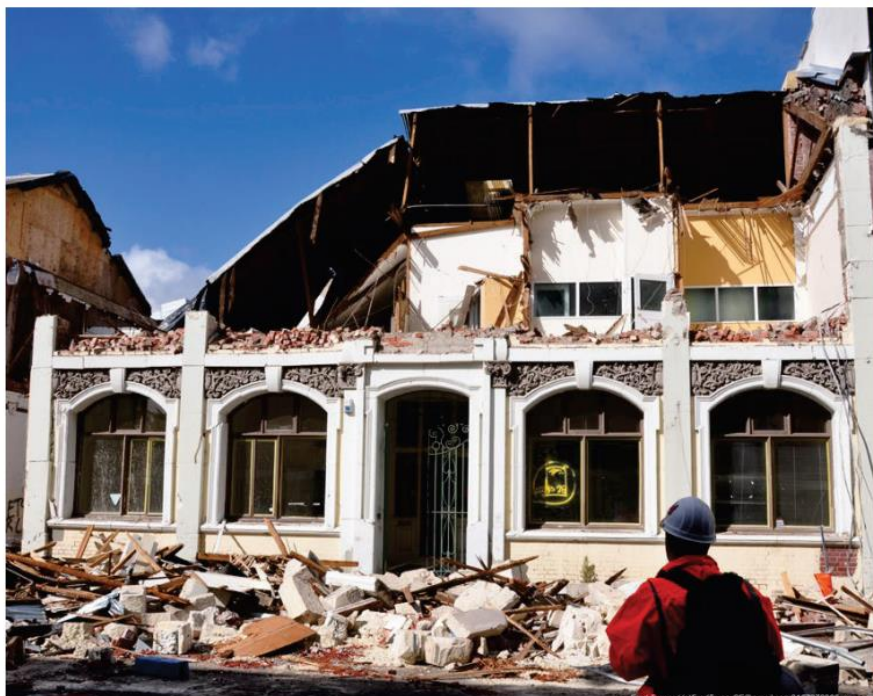
Figure 6-13 Earthquake-damaged unreinforced masonry wall structure in Christchurch, New Zealand (from Fred Turner)
