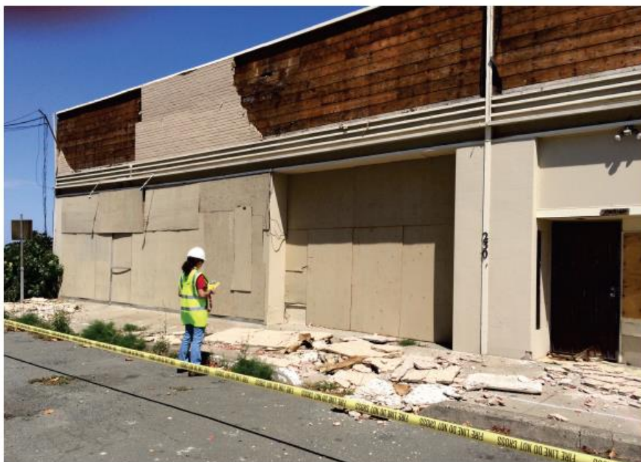
Figure 7-3 Veneer damage in the 2014 South Napa Earthquake (from L Whitehurst, EERI Learning From Earthquakes)
