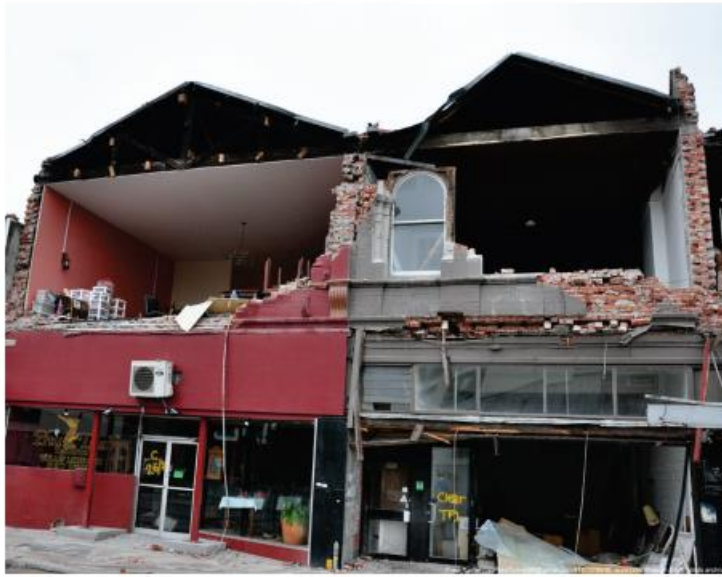
Figure 11-16 Earthquake-damaged unreinforced masonry wall structure in Christchurch, New Zealand (from FEMA P-530).
