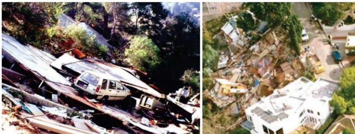
Figure 11-7 Dwellings located on hillside sites and damaged during the Northridge, California, earthquake (from FEMA P-530).
