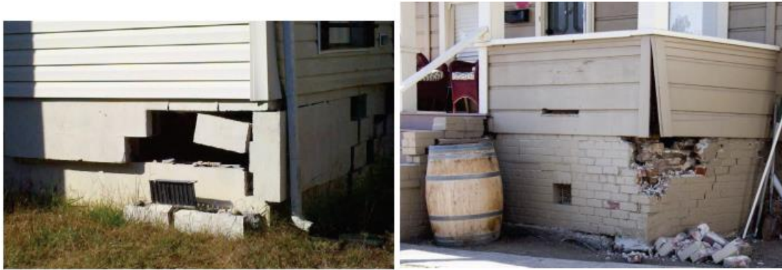
Figure 11-18 Earthquake damage to unreinforced masonry foundations in the 2011 Mineral, Virginia Earthquake (left) and 1994 Northridge Earthquake (right) (from FEMA P-530).
