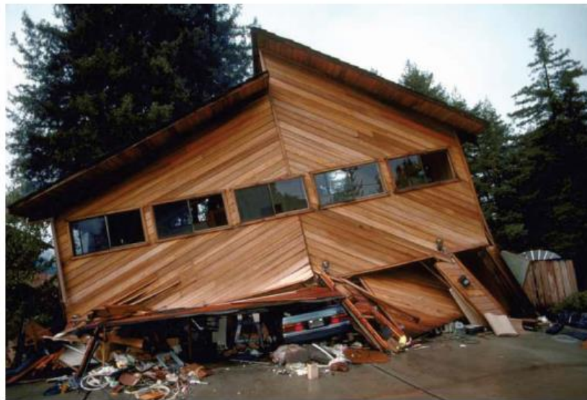
Figure 2-20 House experiencing soft- and weak-story behavior in the 1989 Loma Prieta Earthquake (from USGS).
