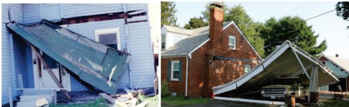
Figure 11-22 Earthquake damage to elevated decks and carports (from FEMA P-530).
