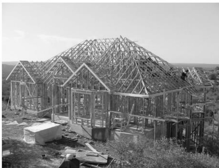
Figure 6-11 Cold-formed steel house under construction (from Dietrich Metal Framing -- a Worthington Industries Company)
