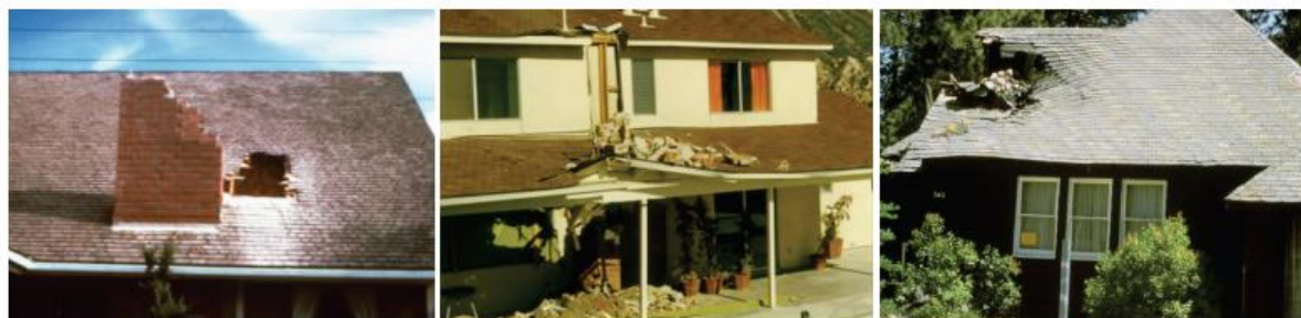
Figure 11-20 Earthquake damage to existing masonry chimneys (from FEMA P-530).
