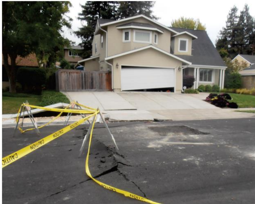
Figure 2-5 A dwelling damaged due to fault movement in the 2014 South Napa Earthquake. (from Geotechnical Extreme Events Reconnaissance, GEER).
