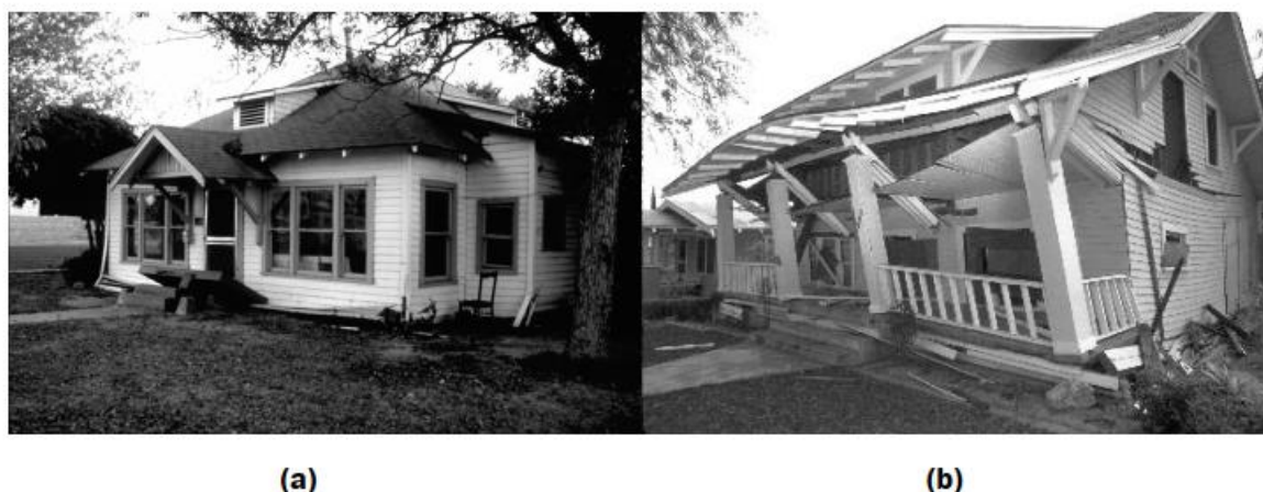
Figure 11-4 (a) House with collapsed cripple walls (from NISEE), and (b) a house with severe damage due to cripple wall collapse (from FEMA).
