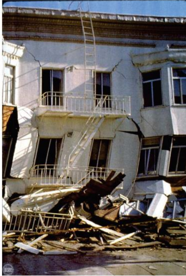
Figure 2-21 Multi-family housing with soft story failure in the 1989 Loma Prieta Earthquake (from NISEE).
