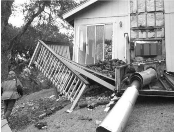
Figure 9-7 Collapsed factory-built chimney, light-frame enclosure, and deck after the San Simeon Earthquake (from J. Marrow).
