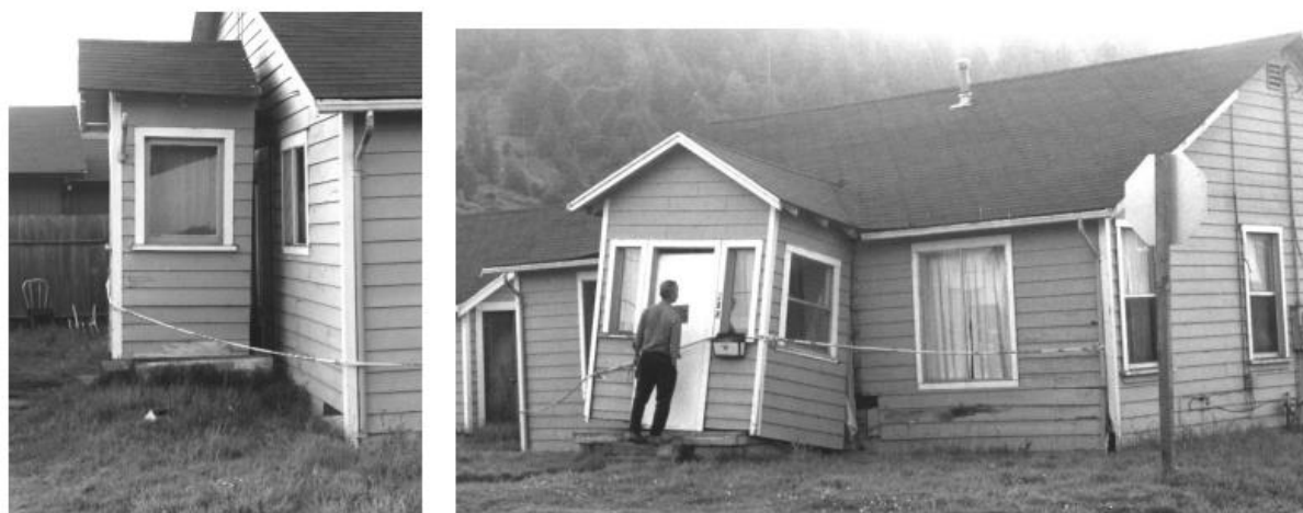
Figure 11-2 Damage to a cripple wall house with slab-on-grade additions in the 1992 Cape Mendocino Earthquake.
