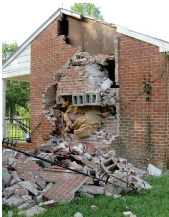
Figure 9-1 Chimney collapse in the 2011 M5.8 Virginia Earthquake (from USGS).
